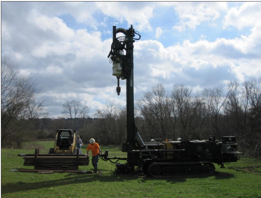
Figure 17 Sonic drill rig mobilizing for a new boring
